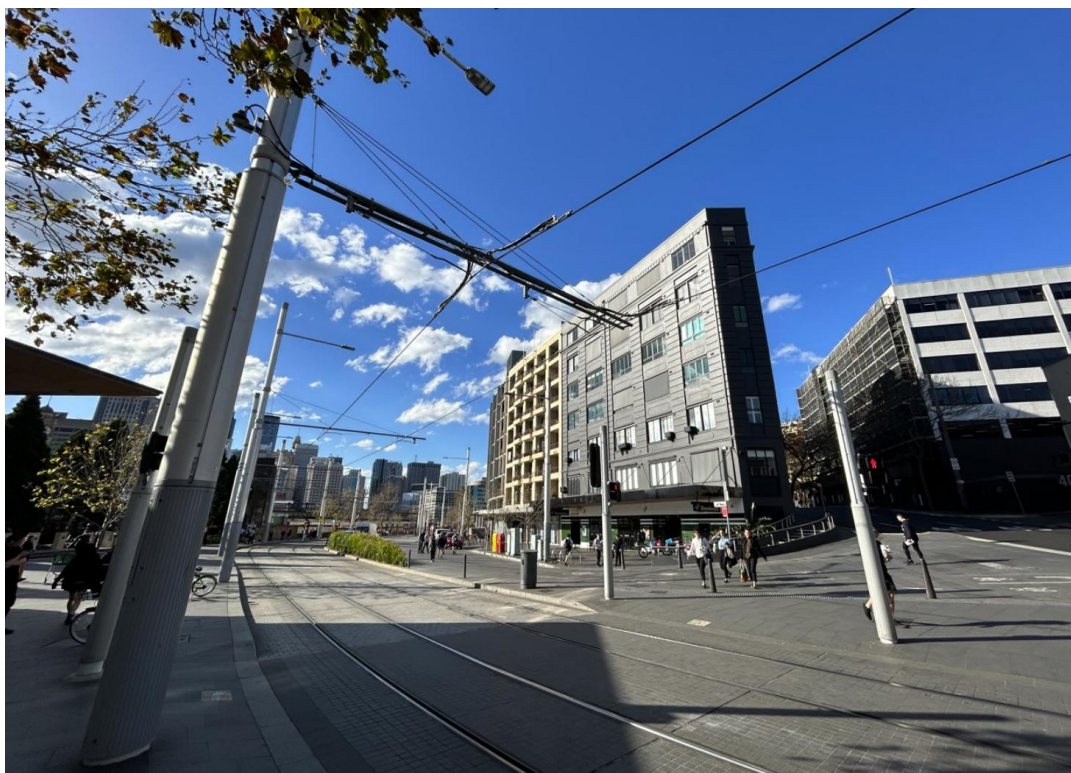
Figure 6 – View of Existing Building – 17 Randle Street from the South with Light Rail Lines in the foreground (Source: City of Sydney)
