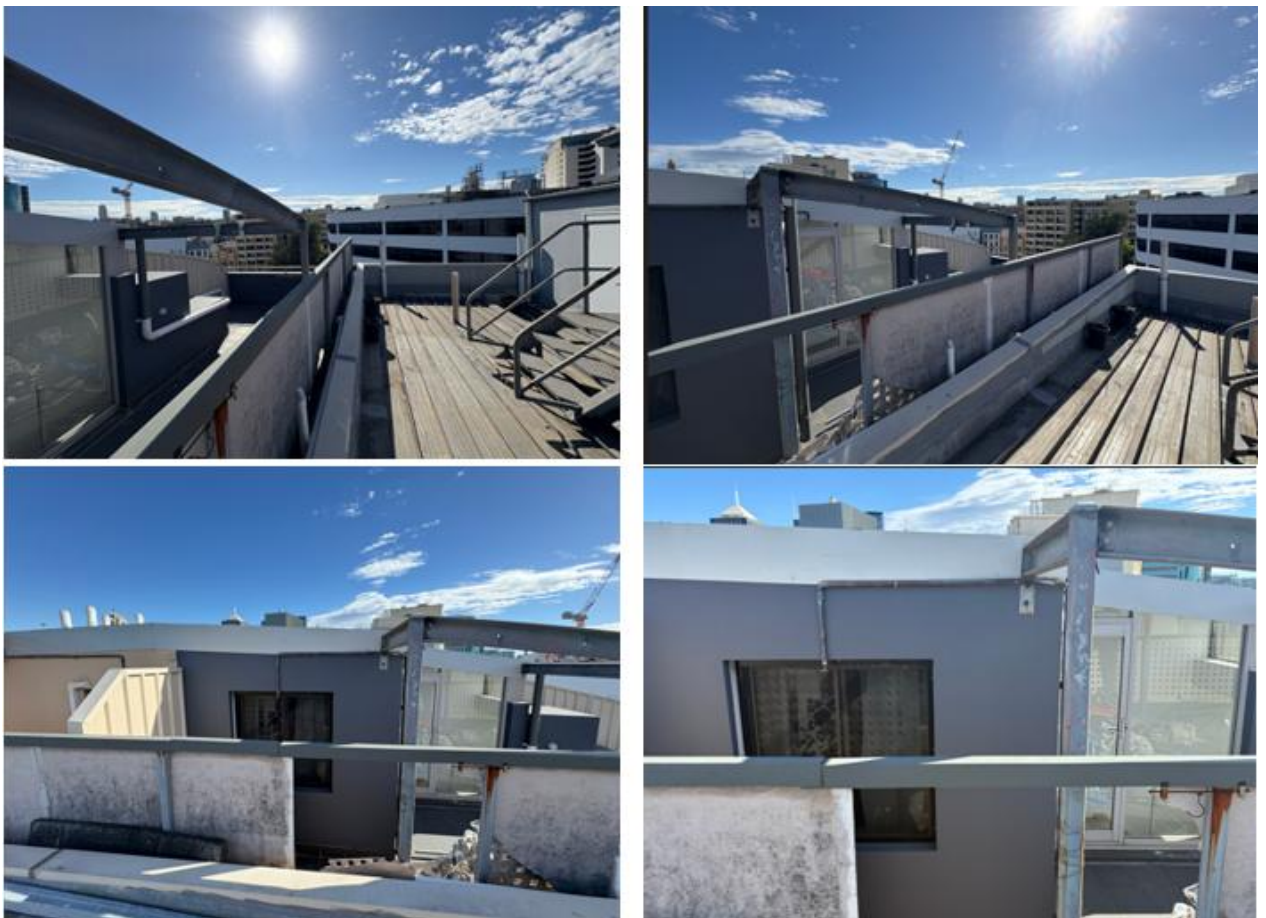
Figure 9 – Photos taken from the existing roof of 17 Randle Street looking toward the common boundary and existing privacy screen located along the boundary of the adjoining roof level apartments of 38 Chalmers Street. (SJB Architects)
