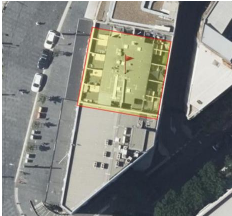
Figure 8 – Aerial view of the roof level residential units and open terraces of 38 Chalmers Street (shaded yellow) and their proximity to the adjoining roof level of 17 Randle Street site (SIX Maps)
